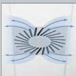
Horizontal two-way air discharge
