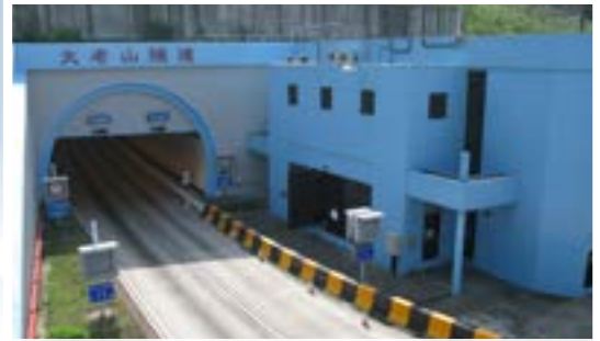
Tate's Cairn Tunnel, Hong Kong
