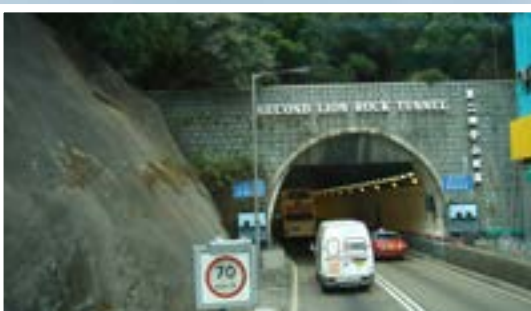
Lion Rock Road Tunnel, Hong Kong
